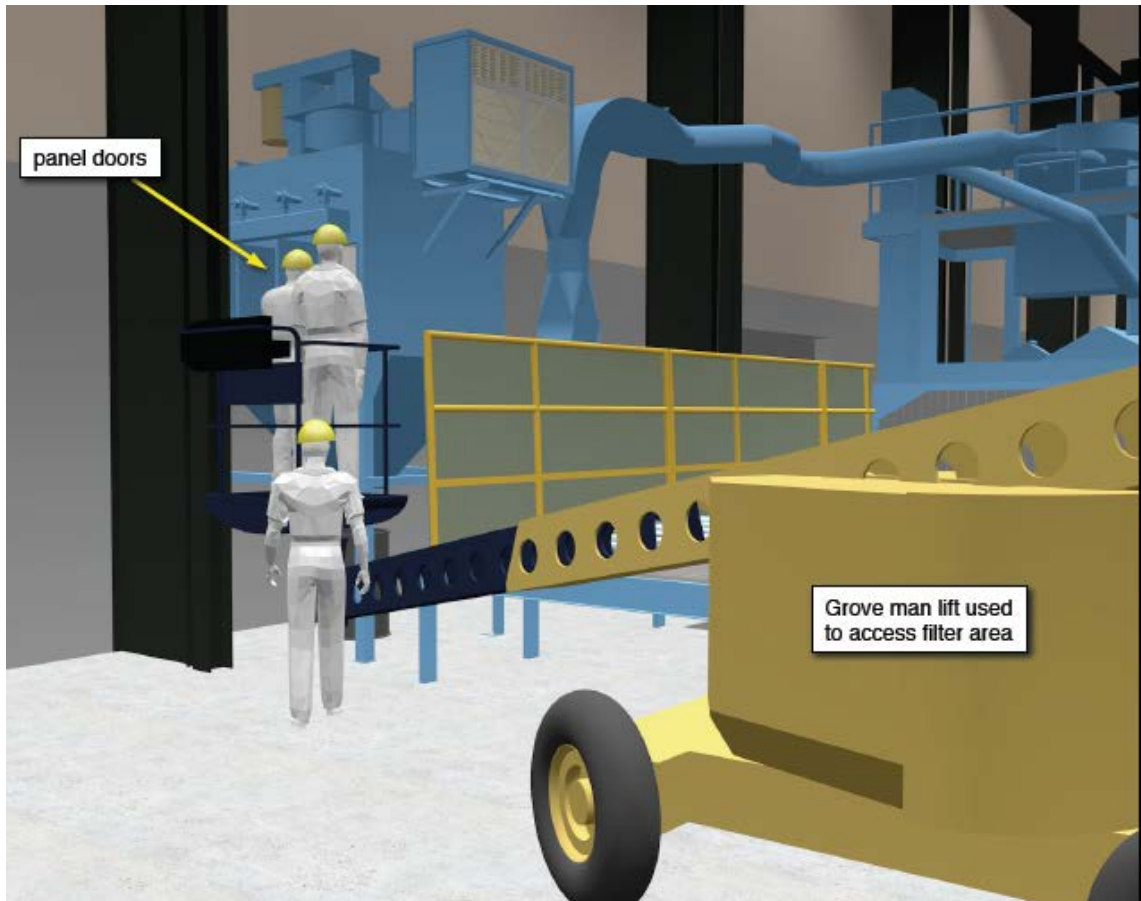
Figure 2. Position of Lift Work Basket and Personnel Next to Dust Collector
